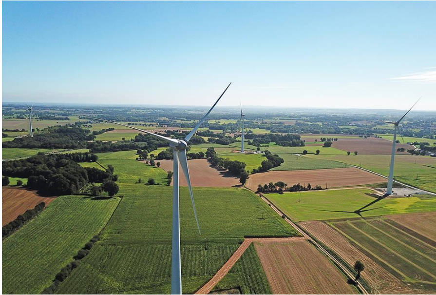
Photo: Broons/Biterne-Sud wind farm
