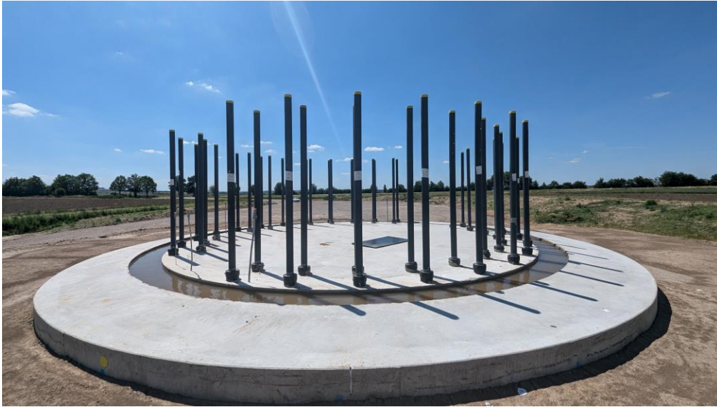
Photo: Foundation of the Enercon turbine E-160
