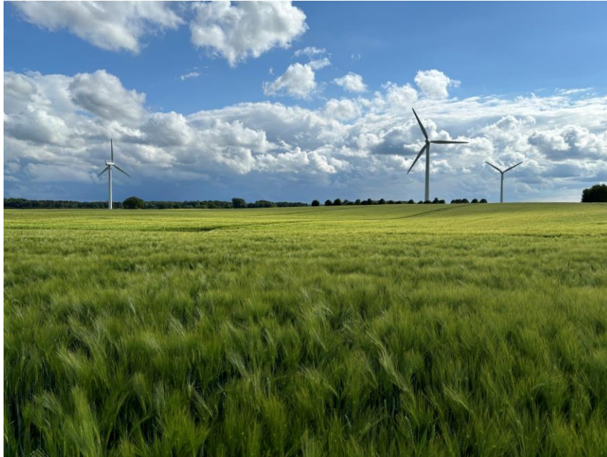
Photo: Section of the wind farm area in Tüttendorf (Copyright: European Energy A/S)
